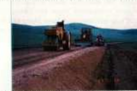
Figure 3.5.7 Compaction and leveling of the subbase course with a motor grader and road roller
