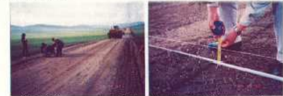
Figure 3.5.8 Measurements of the height of the top of the layer with a leveling string
