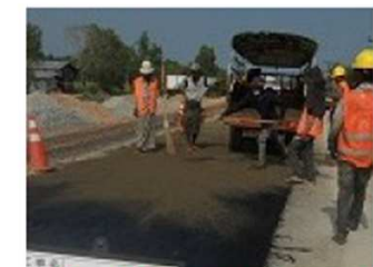
Photo-3.1.29 Spreading curing sand
