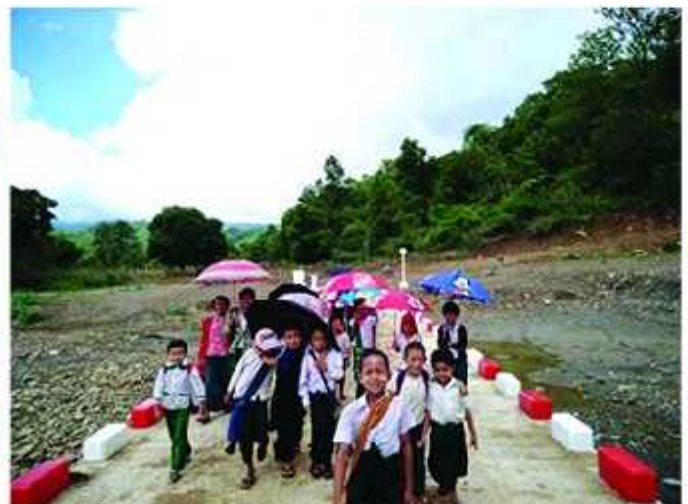
Students crossing the bridge happily.
