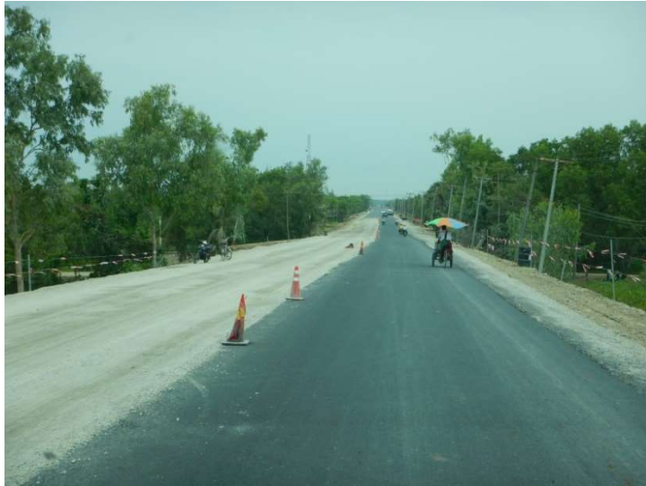
Section where the base layer is paved
