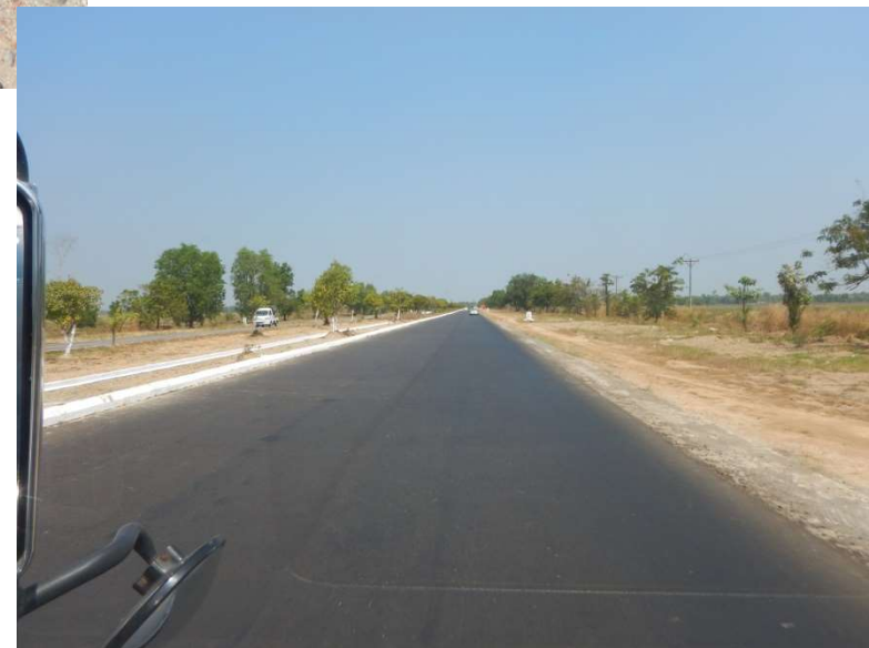
Main line between Pyapon and Yangon The unevenness of the asphalt suggests that it is a PM pavement.
