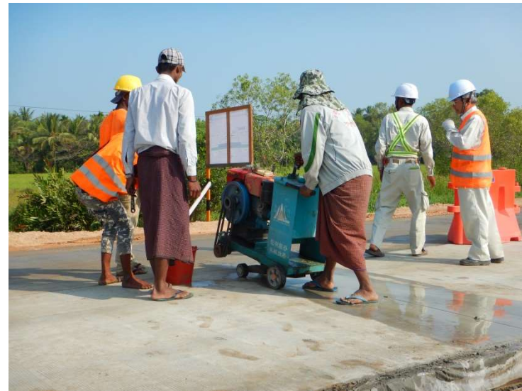
The next day, cutters were inserted into the struck seams and shrinkage joints at a pitch of 5 m.
