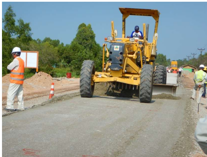
Roadbed leveling operator is MOC staff
