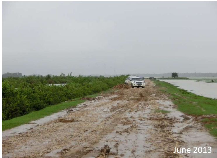
10km south of Pyapon, the road was so muddy that even the Land Cruiser had to turn back. 0-1% CBR?
