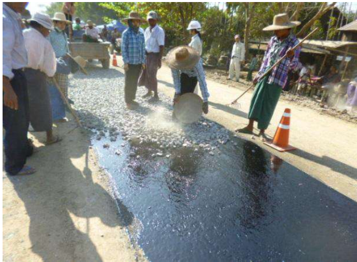
Layer 1 under construction Multilayer surface treated pavement
