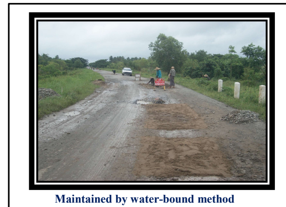
Large crushed stone pavement for PM pavement (left) and repair of damaged road using "water tightening method". (From PPT released by MOC in 2013)
