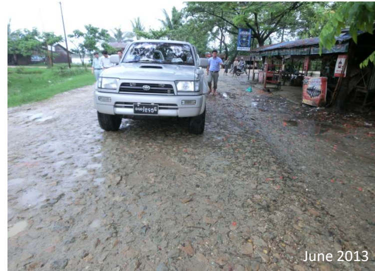
The gravel pavement they call Metal road, a macadam pavement of British origin.
