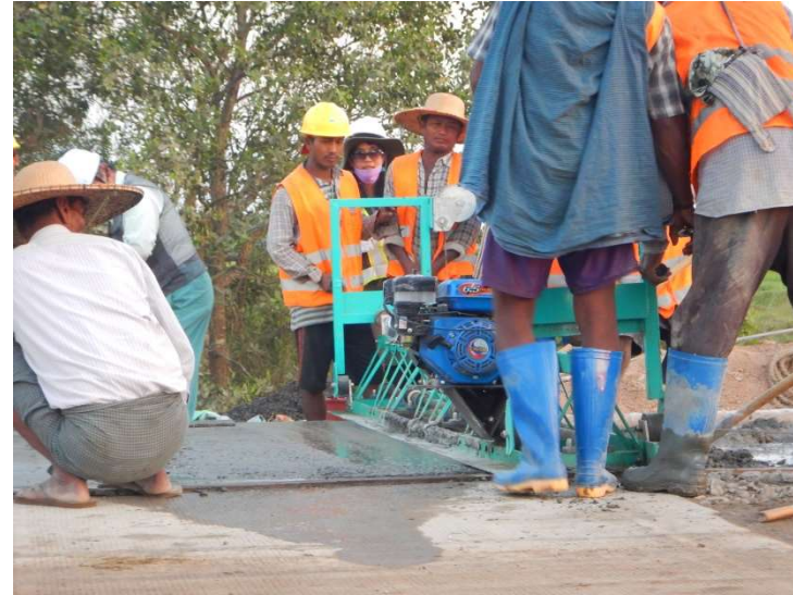
Finishing with a simple finisher
