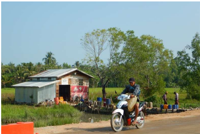
The road body is built with a side-borrow-pit, so the side of the road becomes a canal. The photo shows gas station.
