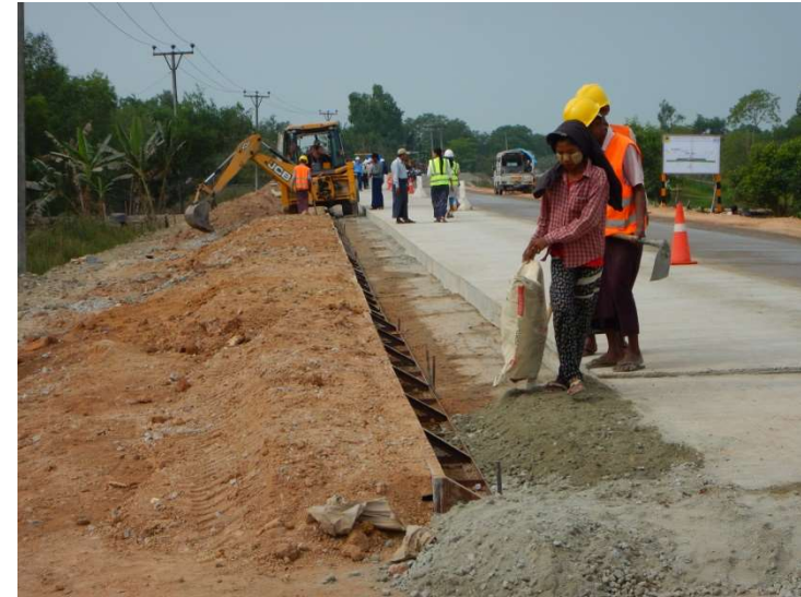
Putting good quality material (crushed stone) on the shoulder (1.2m width). Cement bags are used as transport containers.
