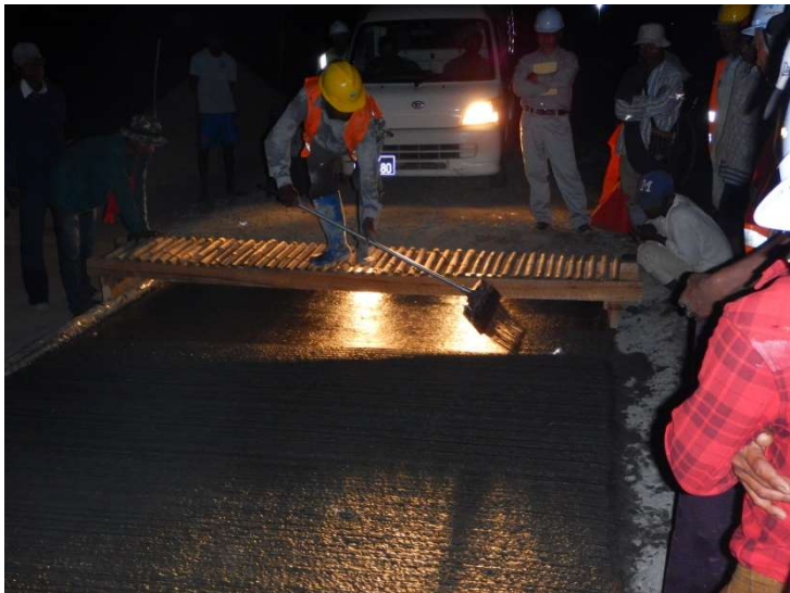
Hand-made brooms were used for broom seeding, and the work took a long time and was done at night.
