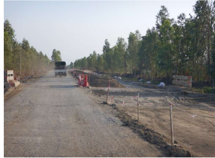
Cement or lime stabilization of the roadbed in progress
