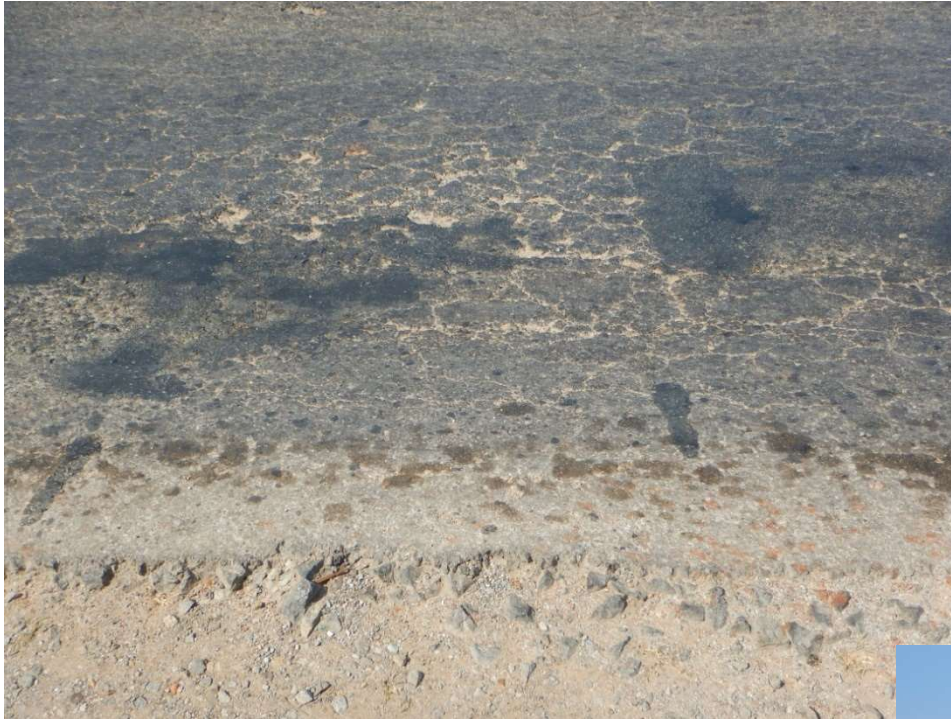
Main line between Pyapon and Yangon The unevenness of the asphalt suggests that it is a PM pavement.
