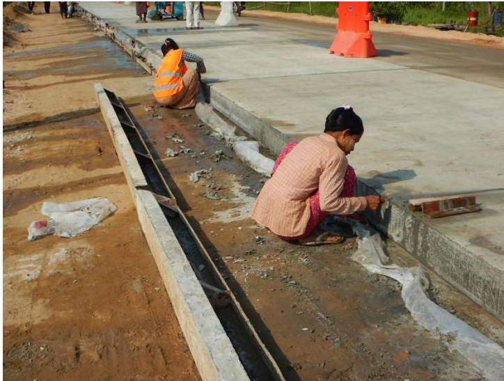
After curing for about a week, the formwork is removed and the shoulder construction is prepared.
